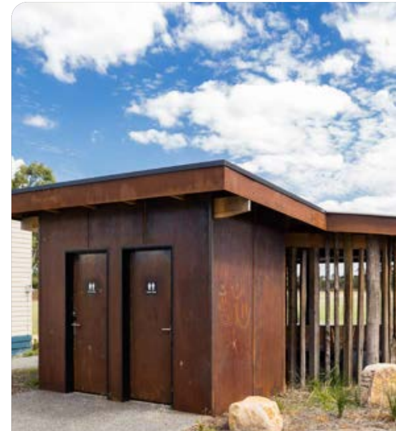
Toilets integrated into an outdoor learning space at an independent school in Victoria. Designer: Cley Studio Photo credit: Peter Casamento
