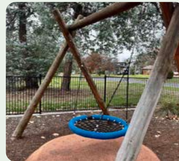
Basket swings with two-point suspension lines restrict movement to a single back-and-forth direction. Photo credit: Marta Day
