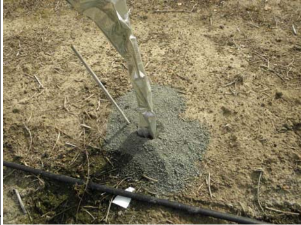
Fig 18. Crusher dust placed around the base of the tree. As the tree moved on the wind the dust falls down the hole alongside the trunk locking the tree in place and providing stability
