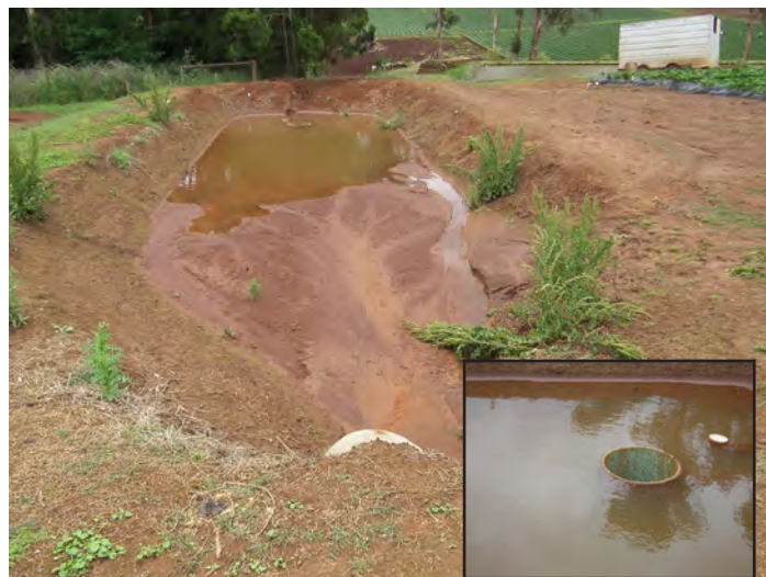
The sediment pond settling out suspended sediments in the water before overflowing through the outlet pipe (insert)
