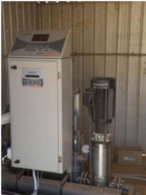
Irrigation controller. Photo: DAFWA
