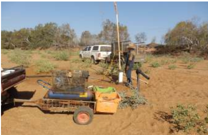
Cleaning out Gascoyne Research Station bore. Photo: DAFWA
