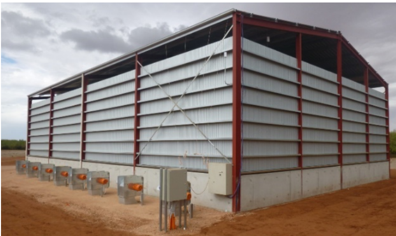
Figure 7. Shed with aerated floor used for drying and rewetting of almonds at Bunyip Reach, Murtho
