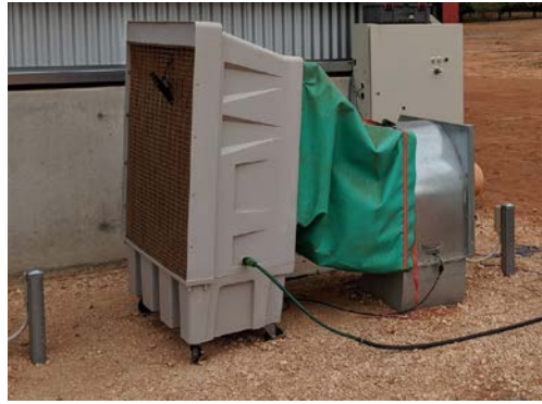
Figure 11. Evaporative cooler added to the fan inlet at Bunyip Reach, Murtho
