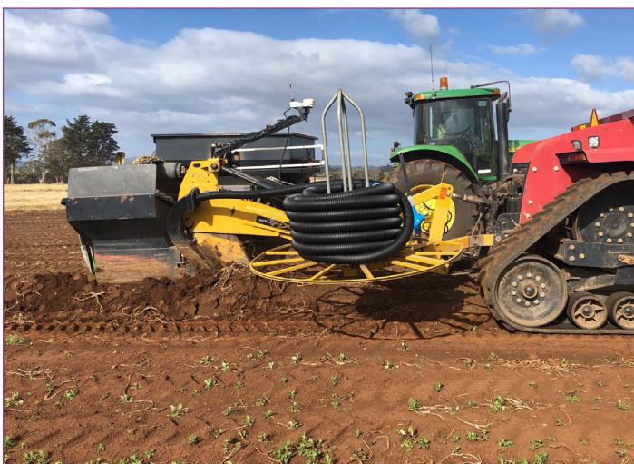
Figure 2. Subsurface drainage installation in progress at ‘Lornebrook’.
