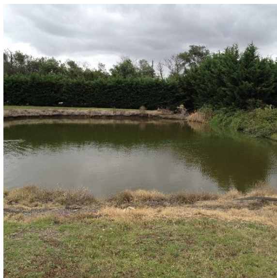
Holding dam for run-off that can be pumped back to the irrigation channel for reuse.
