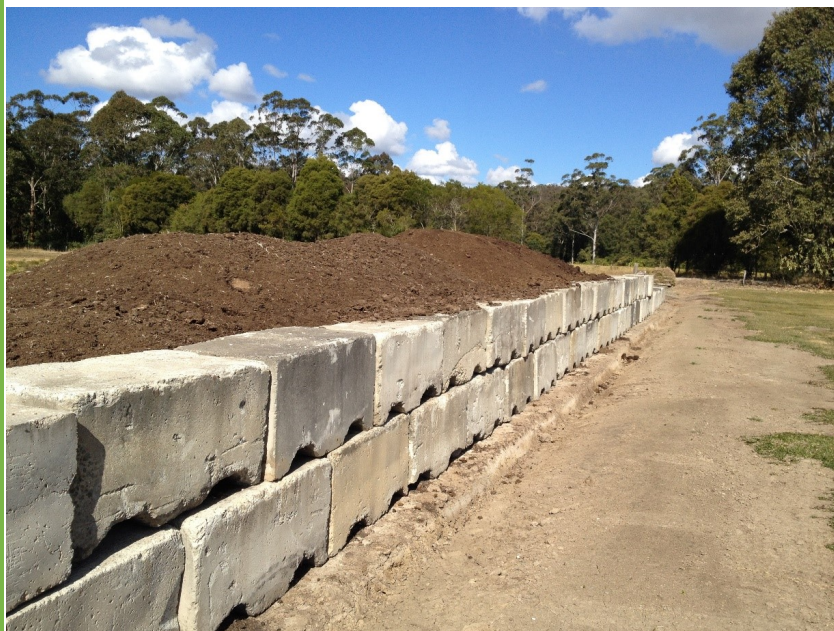
Agland's retaining wall around a manure pile saves most of the wind-blown and run off losses
