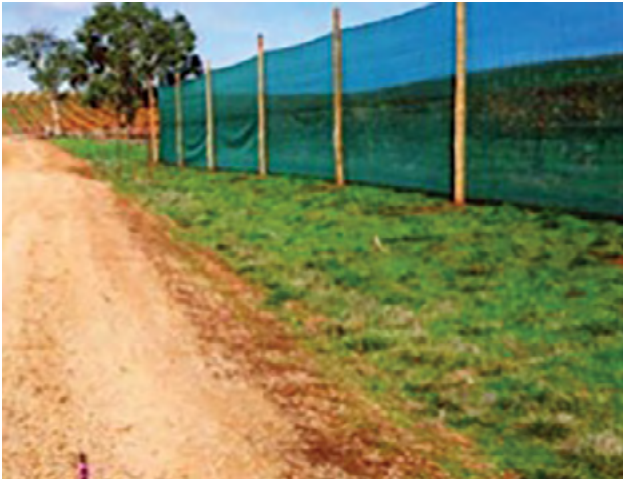
Figure 10. An artificial barrier made of shade cloth with 50% porosity. Photo: Andrew Hewitt.
