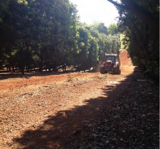
A row of trees has been removed and the ground is being shaped for an interrow drain.
