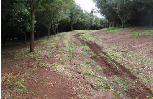
Trees were removed to create this graded bank in an established orchard.
