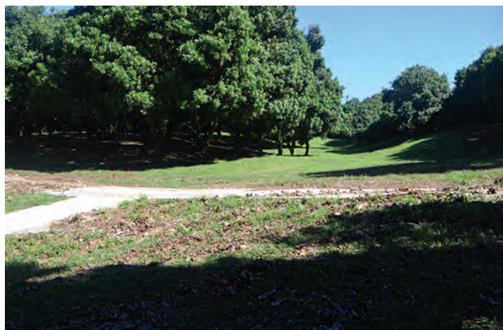
Some concrete was used to allow an access road to cross this grassed watercourse. The trafficked pathway had been scouring out, needing more than grass cover to protect it.
