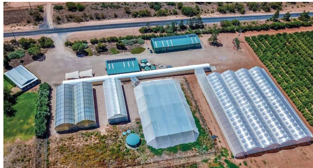
A drone image of the new facility.
