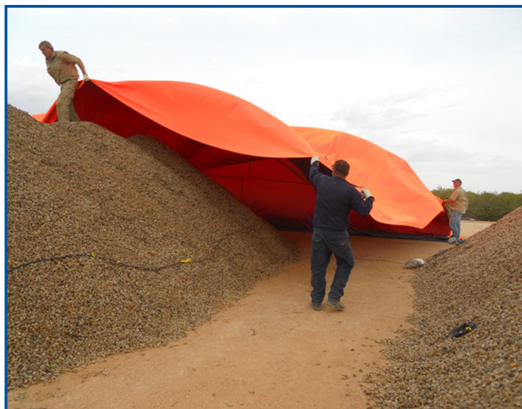
Figure 5. Covering stockpile with a breathable, waterproof tarp.
