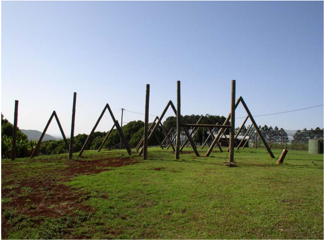
Block with all support poles in place
