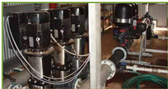
The new pumping, fertigation and filtering system. Row spacing allows for mechanical harvesting
