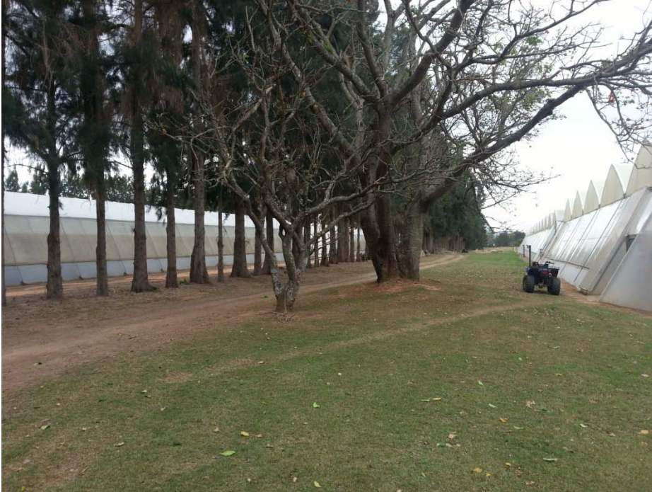
Figure 1: external view of screenhouses
