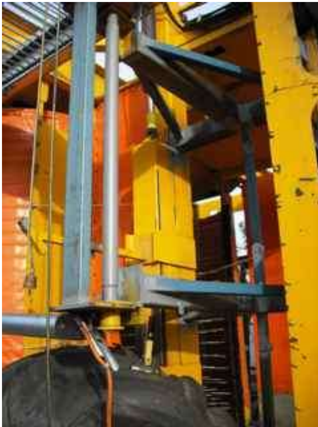
Photo 8 – Strengthen main frame to carry overhead conveyor.
