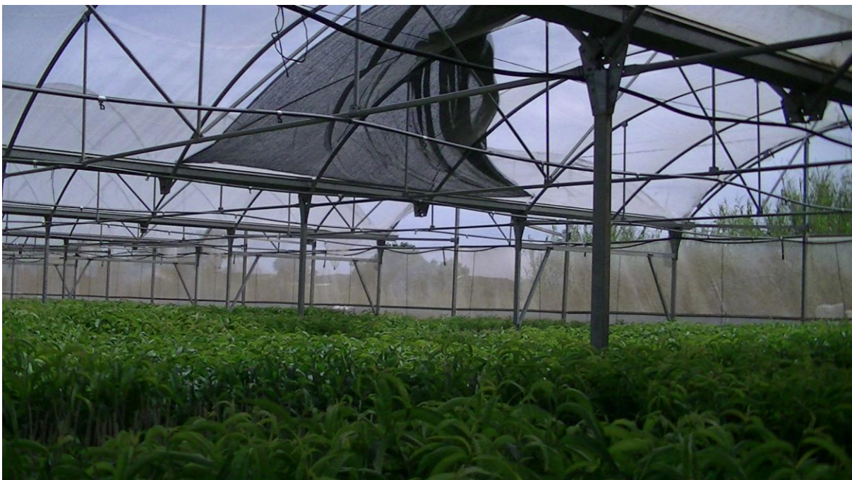
Figure 2: Shade house structure and spray irrigation at elviverodeabel nursery, Caspe, Zaragoza.
