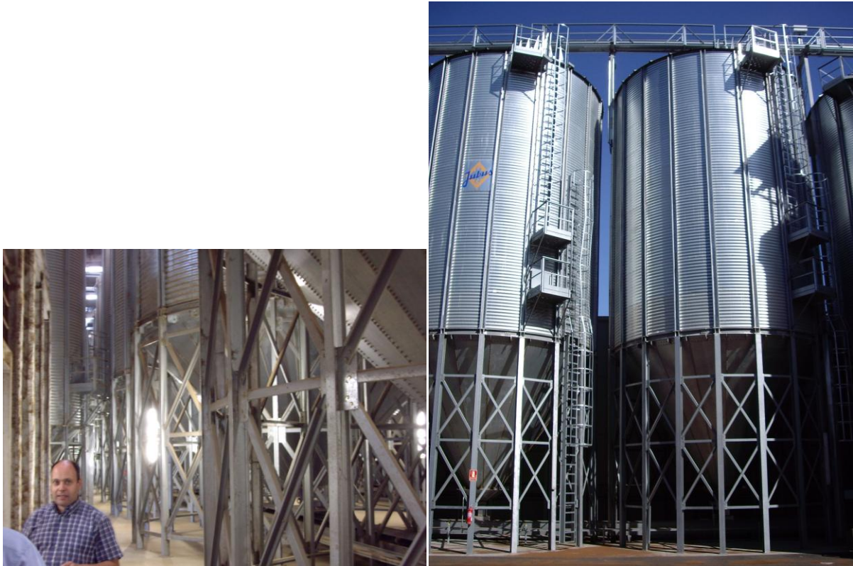
Figure 20: Controlled climate silos for storage of in-shell product awaiting shelling, or raw kernel, UNIO Almond Corporation, Reus, Spain.
