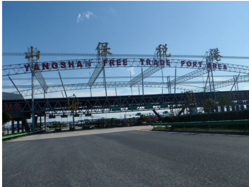
Entry to the Port facility
