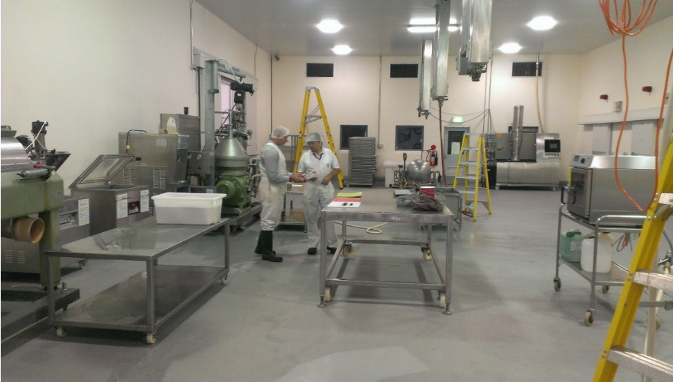
Figure 7. CSIRO Pilot Plant facilities.
