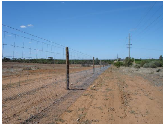
Figure 4 Fence surrounding property
