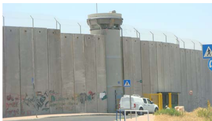
above- the wall between Israel and the West Bank in Jerusalem.
