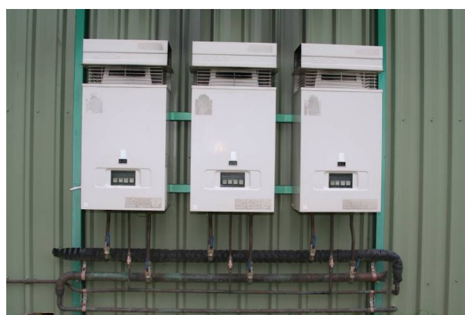
Plate 22 The gas-fired heating system for the hot spray unit.
