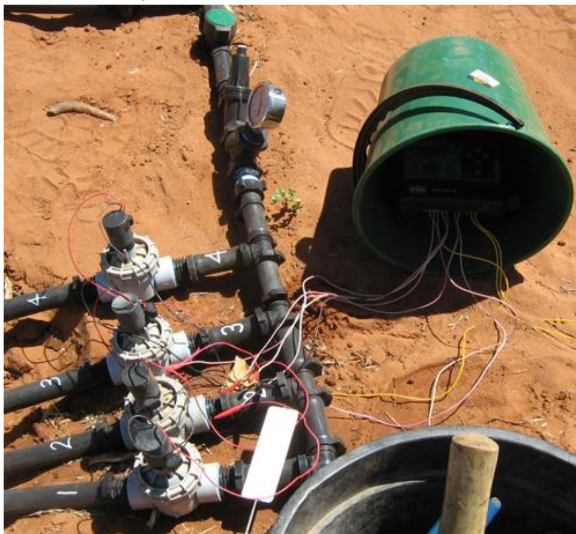
Photo 10.1 – BC0902: Complex installation, required four separate controllers providing four independent watering lines to the four different treatments.
