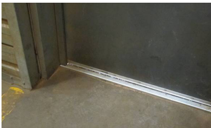
Figure 9. Small holes (>6 mm) allow entry by mice into sheds and facilities. This is especially important on the edges of roller doors, where it is difficult to reduce the gaps. Top: a small gap along the side of a roller door will allow access by mice into the facility. Bottom: well-fitting metal door strips will stop mice entering the facility.
