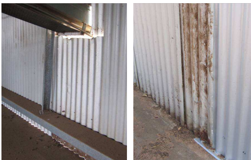
Figure 18. Left: If mice can grab hold of the edge of corrugated iron, they can climb up and climb through small gaps around elevators such as this. Right: Mice can climb up poorly fitting wall panels. These need to be fitted together with no overhang.
