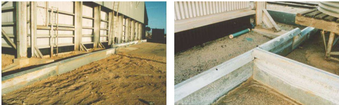
Figure 9. Mouse-proof fence at a grain silo in Victoria. A bait station (PVC tube) is pictured on the right, inside the fence in case mice gain entry.
